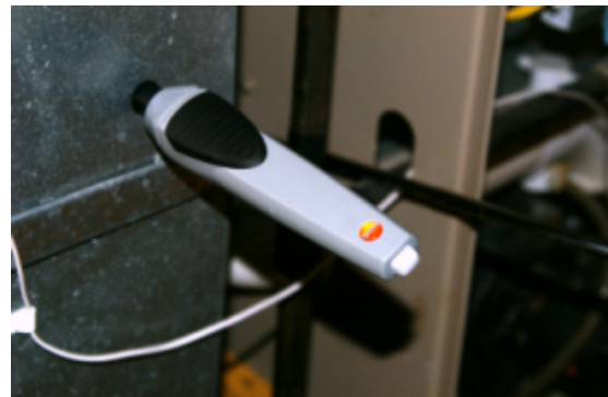
Wireless probe located in the return
