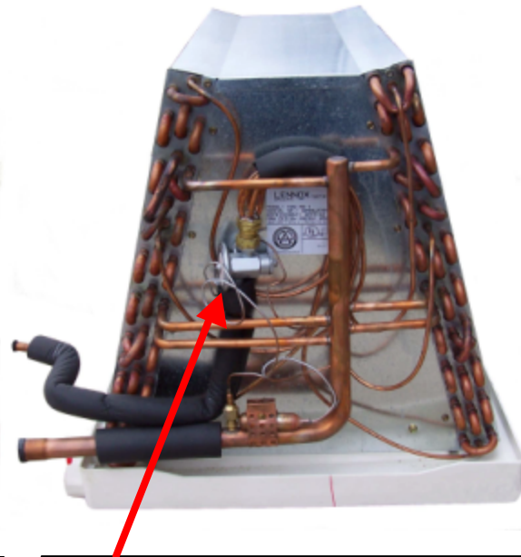
Thermostatic Expansion Valve (TXV)
