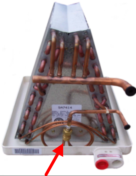
Fixed Metering Device Short Orifice
